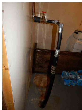
Water line into house comes into cold room
